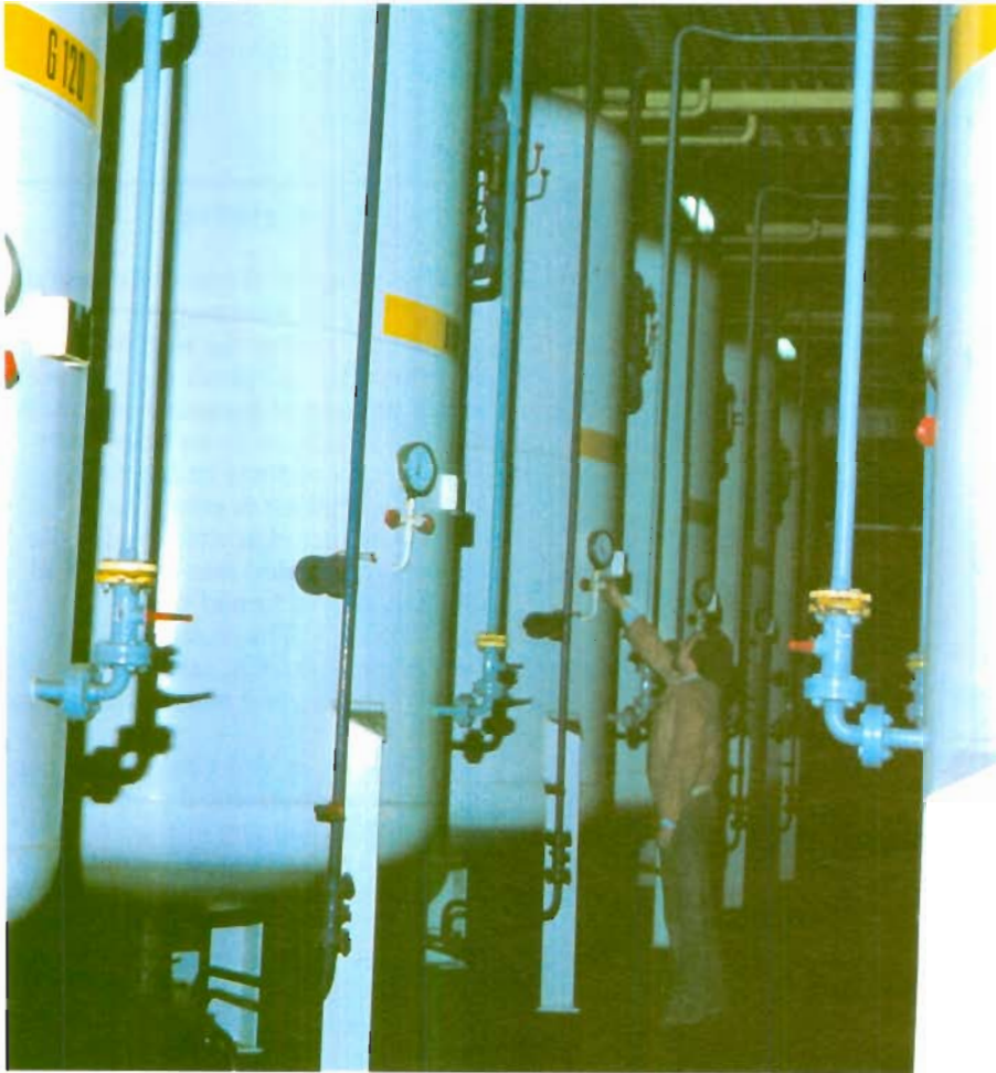
A worker is dwarfed by the storage tanks which hold the mixed test gases used by the Gasinstituut. The test gases are used for studying performance of gas burners and as GC calibration samples.
